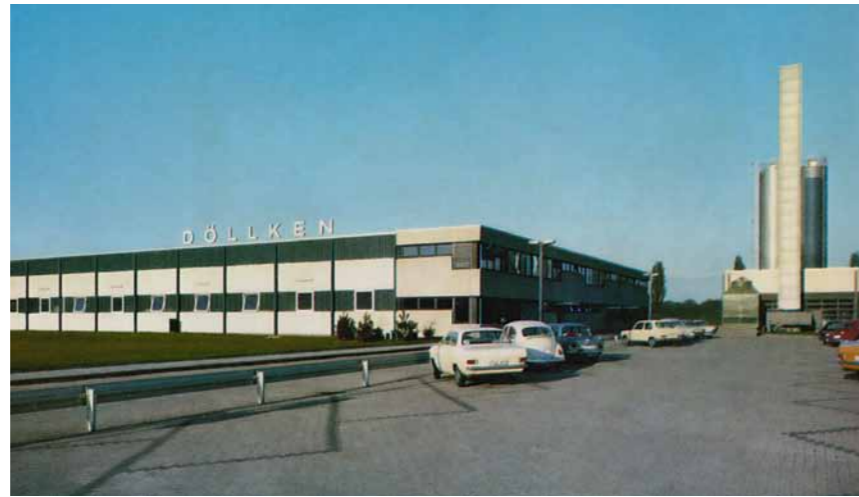
Plastics plant II in Gladbeck brings new capacities
